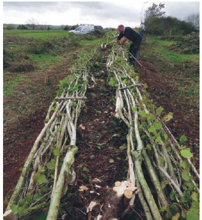
Here the steepers have been placed along the edges of the bank top by Mike Reed and Russell Woodham, leaving the centre clear, to create a double comb. ©Robert Wolton
