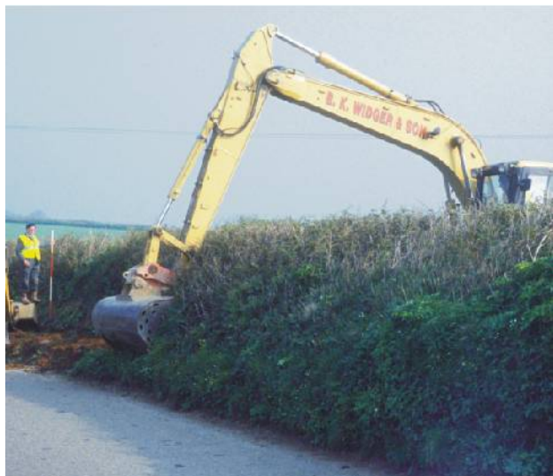
Figure 4: Use the excavator bucket to cut into the side of the hedge facing away from the direction of movement. ©Peter Chamberlain
