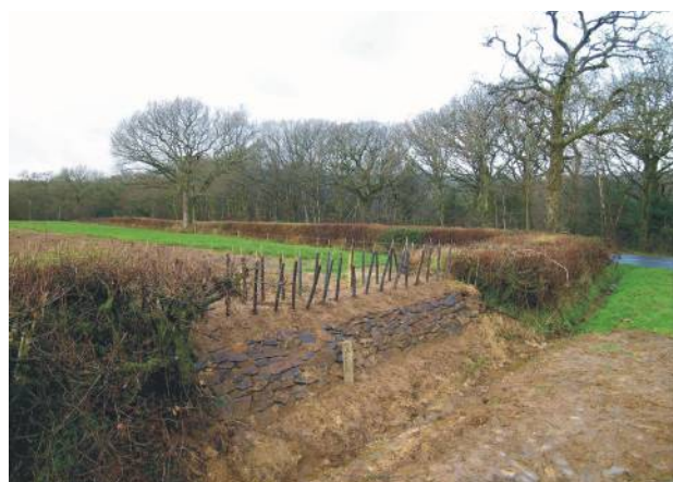
Although this section of reinstated bank is of similar dimensions to the original, there was no stone facing to begin with and the bank is taking a long time to blend in. Turf facing would have been better. The young shrubs (whips) do not mirror the species mix on either side, and were slot planted: establishment has been poor. ©Robert Wolton
