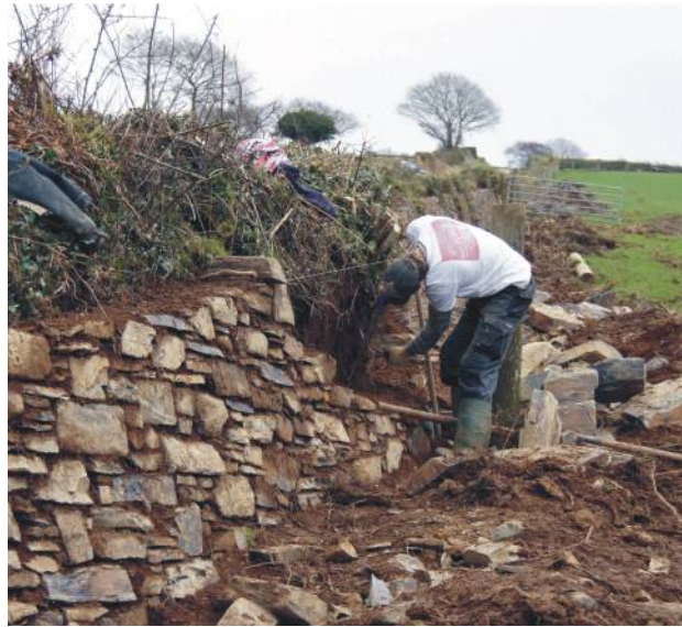
Repairing stone facing. ©Robert Wolton
