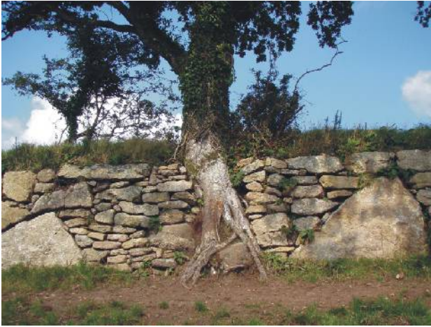
The stone faced bank on either side of this oak has recently been restored. ©Stephanie Knight
