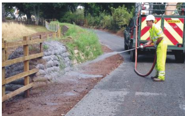
Figure 5: Hydroseeding the surface of hessian sacks. ©Paul Couttie
