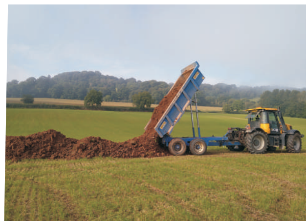
Soil from the creation of shallow ponds (scrapes) in a floodplain just 100m away is being used here to create a new bank. Photo Simeon Day.
