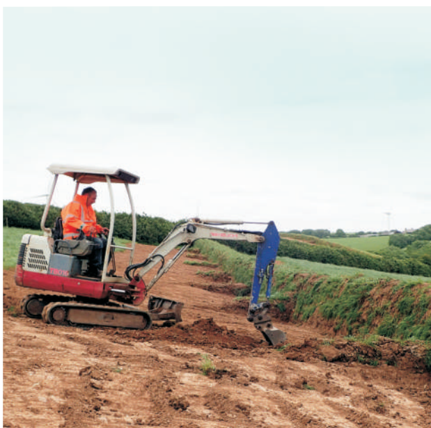
A new hedge being made along a contour to reduce flood risk further down the catchment.
