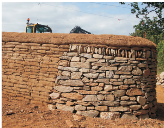
Reinstatement of a massive hedge bank using stone-facing and hessian netting and bags.
